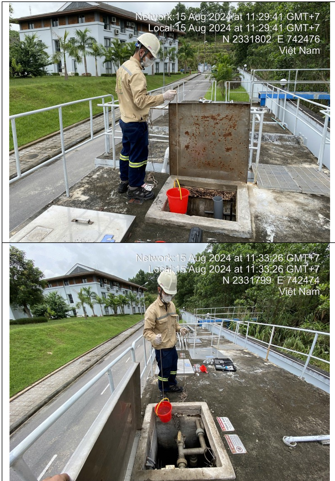
Figure 4.6. Sampling sanitary wastewater in the housing colony area
