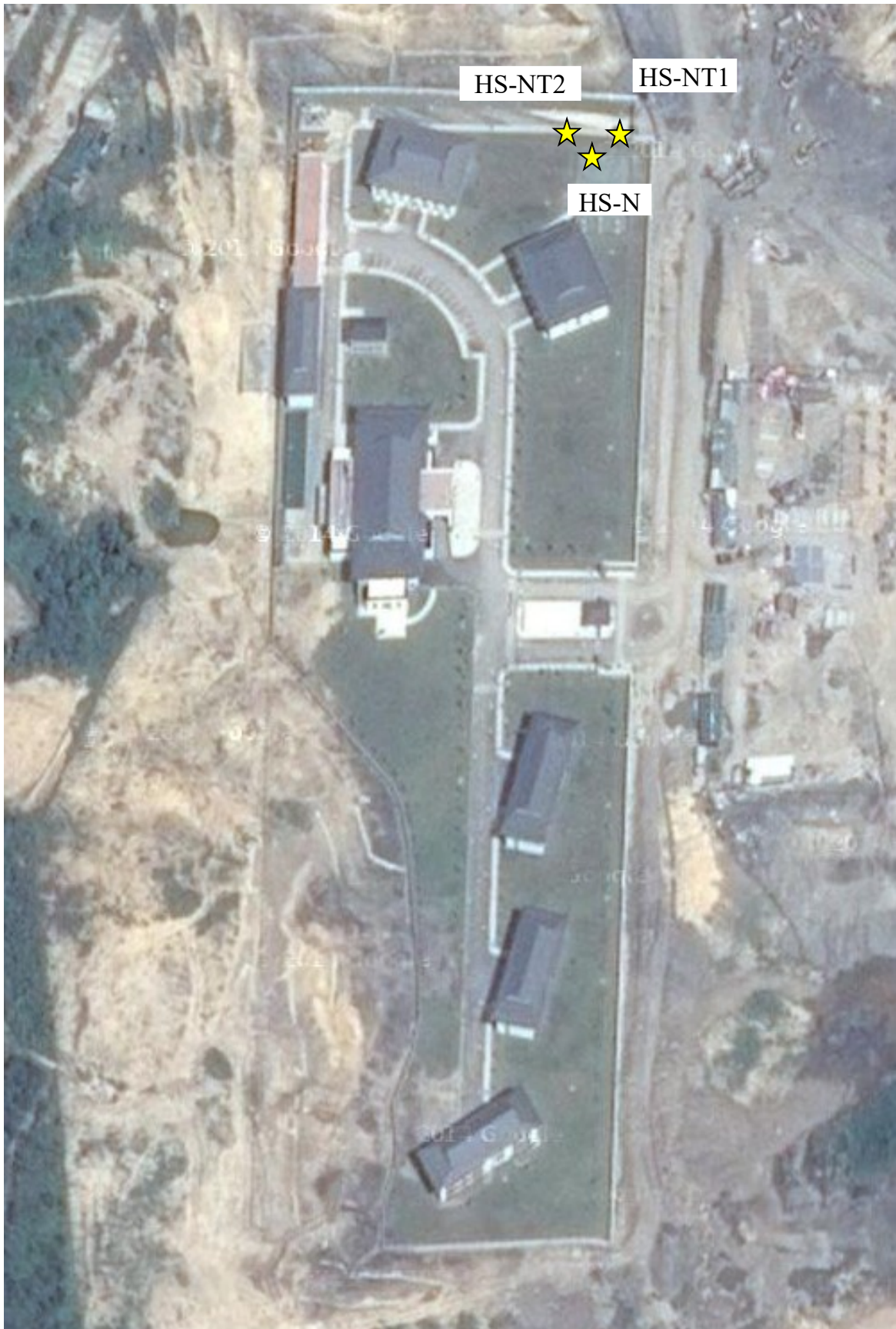
Figure 4.10. Wastewater sampling positions
