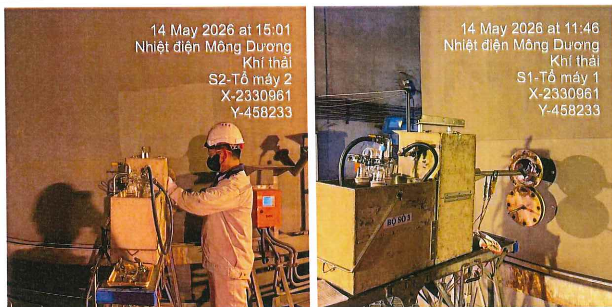
Figure 4.3. Air emission sampling in the plant
